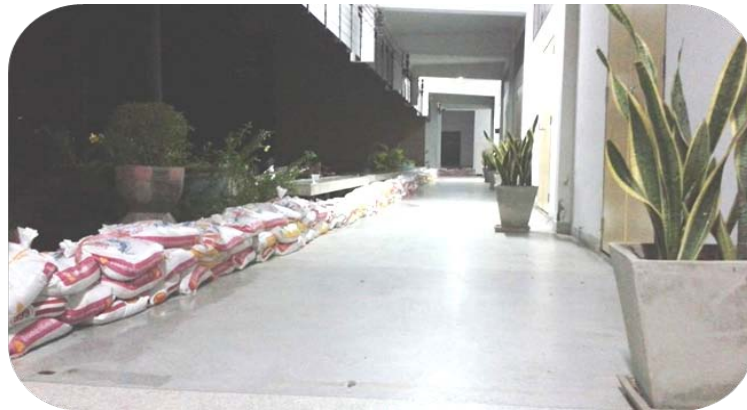
Figure 5: Current flood protection by using a sandbag dike.
